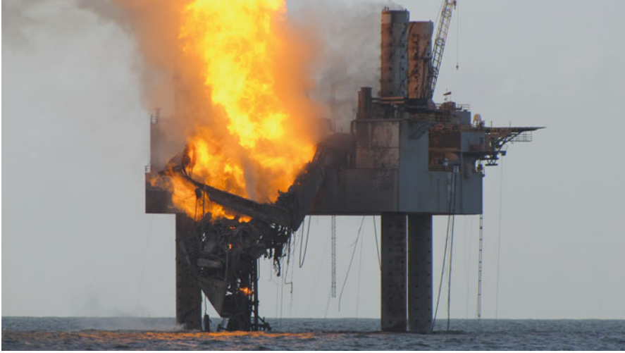
Fig. 6 The Hercules 265 natural gas drilling platform was on fire several days before collapsing. Photograph from the U.S. Coast Guard
